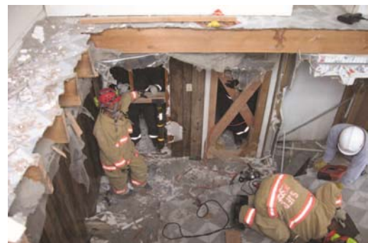
Crews train to respond to building damage caused by earthquakes.
